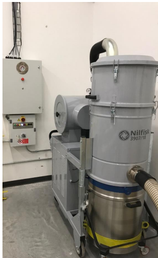
Central Vacuum System
